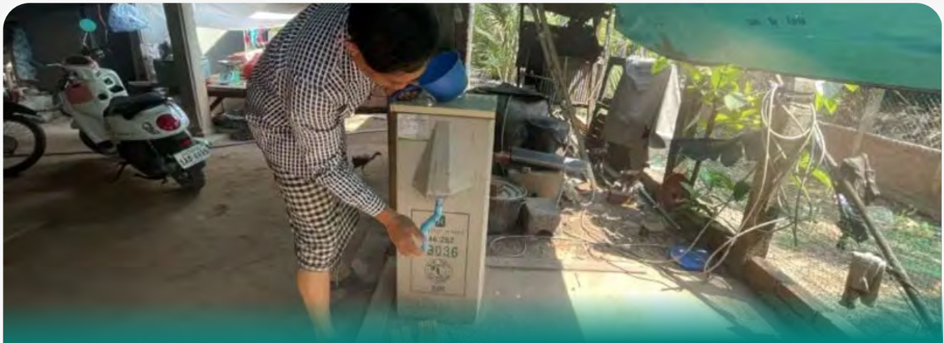
Vireak shows how the sand filtration system works. However, it is not effective in removing contaminants, hence an urgent need for reliable and safe drinking water solutions. Photo taken on March 23, 2025. (Eung Sea)
